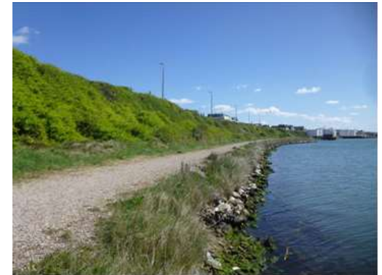
North Canal Bank
