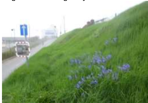
Basin Road North embankment
